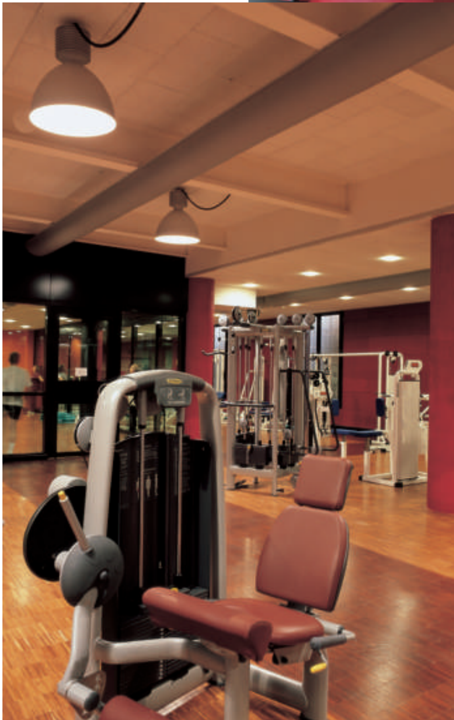
Zone cardiofitness e circuit – training - Rivestimento soffitto in sughero SoKoVerd.C1
